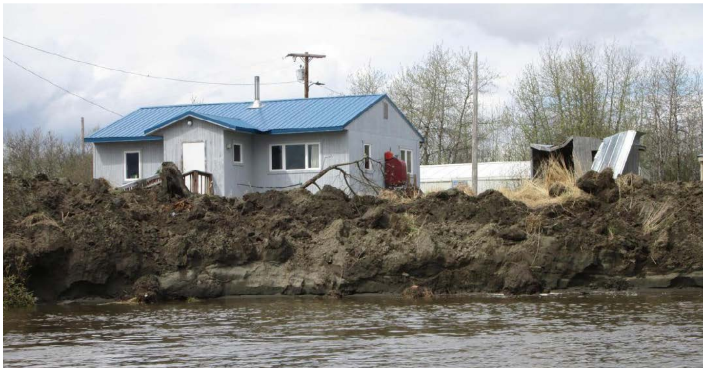
Figure 12: Rapid erosion in Akiak claimed 50-75 feet of riverbank over two days. Credit: Ivan Ivan
