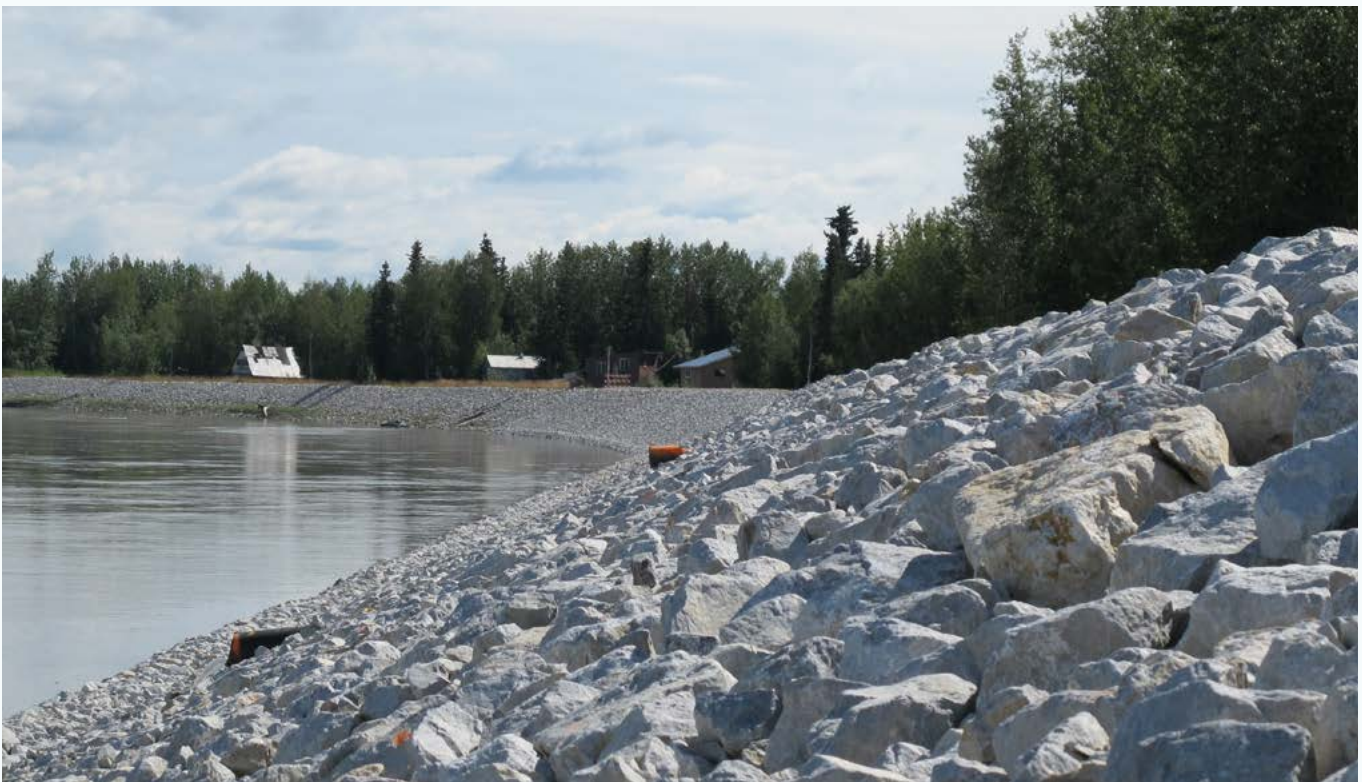
Figure 45: Armored riverbank at McGrath. Credit: Natural Resources Conservation Service; 2015.
