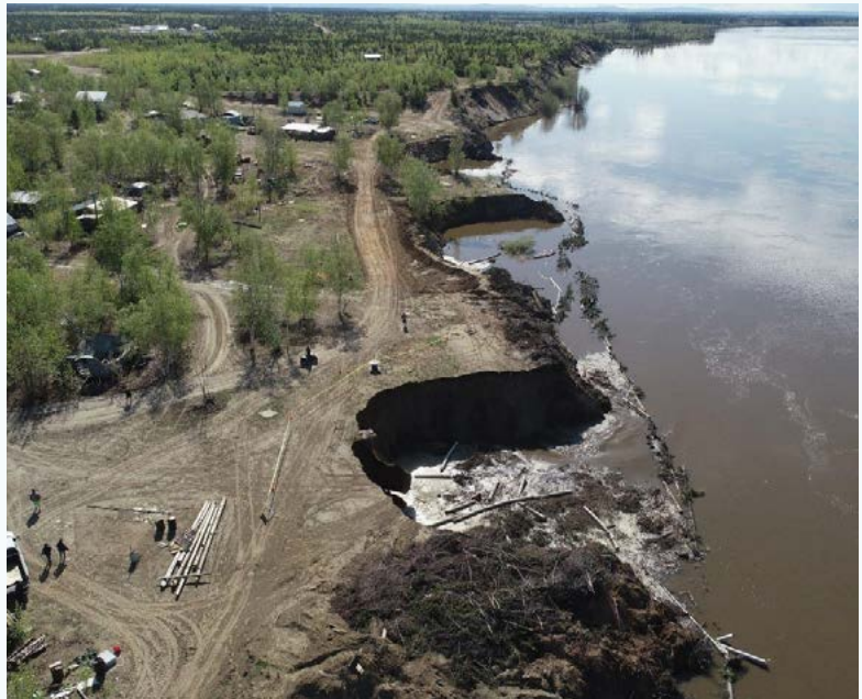
Figure 46: In 2018, sections of the riverbank in Huslia were lost to rapid erosion. Credit: Huslia Village; 2018.
